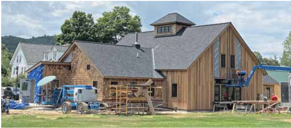
The Proctor Woodlands Building is nearing completion. The final project in the $40M+ Campaign for Proctor, the Woodlands Building will serve as a science teaching space and gateway to Proctor's 2,500 acres of woodlands. The timber frame construction of the building utilizes timbers harvested on Proctor's land near Elbow Pond. Caption and photo: Scott Allenby
