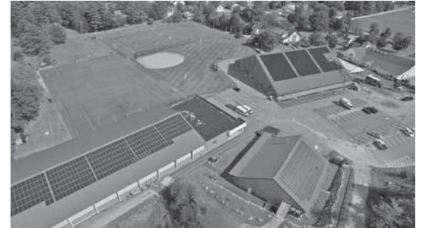
Proctor Academy completed the installation of its 11th solar array this summer, a one acre, 412,000 kwh array on the Farrell Field House.
